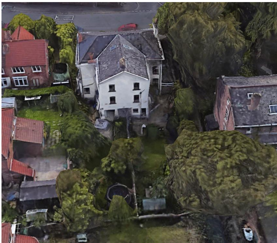
View of the rear of the application property to the right and adjoining semi-detached property
