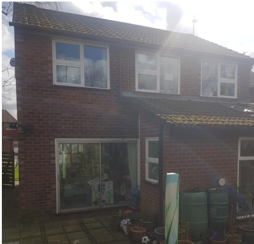
Rear view of No.25 Hampton Road
