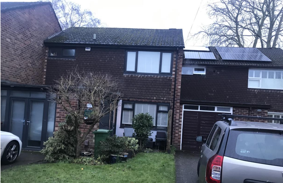
Front view of No's 23 and 25 Hampton Road
